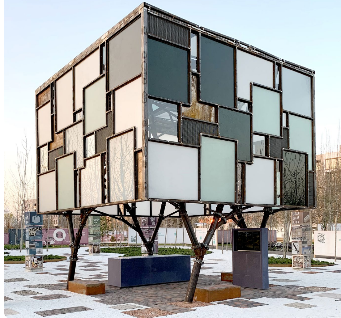
The Mehr.WERT.Pavillon at the German Federal Garden Show in Heilbronn, southwestern Germany, 2019. It uses recycled glass, steel from a dismantled coal-fired power plant, broken concrete, and porcelain. Courtesy of Felix Heisel.
