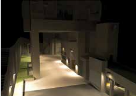
Image courtesy of Hong Kong Housing Authority
