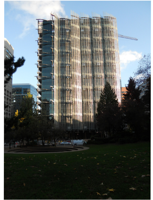
System of shading "reeds" on west side of building. Image courtesy of SERA Architects.
