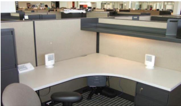
Figure 2. Johnson Controls Personal Environment Module with occupant sensor, control panel (on left), integrated task-light and desktop vents from underfloor air supply.
