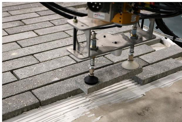
**Fig. 6** Placing a cladding module in the assembly. Placement targets are calculated on the fly based on the assembly progress thus far and the dimensions of the material in hand
