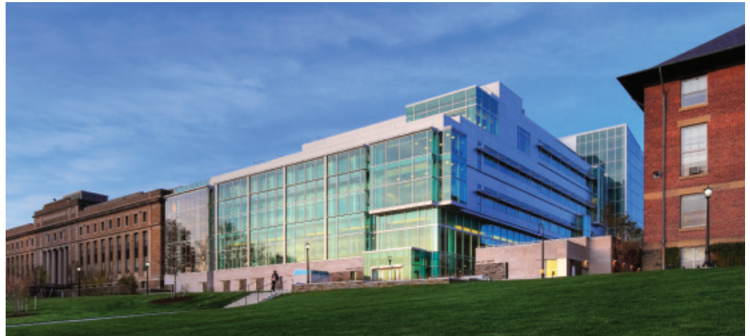
Image courtesy of McCarthy Building Companies, Inc.
