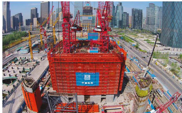
The Intelligent Construction Equipment Integration Platform was developed by China Construction Third Engineering Bureau Group Co., Ltd. It is 22m in height, its gross area exceeds 1,800m 2 , and has the highest loading capacity in the world. With the assistance of this platform, one single structural floor can be completed in three days. Image courtesy of China Construction Third Engineering Bureau Group Co., Ltd.
