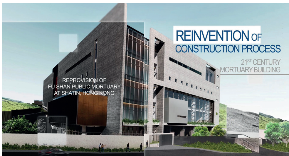
From BIM to DfMA: the reinvention of construction process of 21 st century mortuary building Image Courtesy of Architectural Services Department, HKSAR Government (ArchSD)
