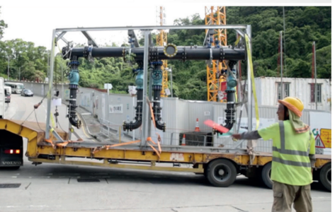
Standardization and DfMA of MEP modules enhances buildability, reduces time, cost and labour. Image Courtesy of ArchSD
