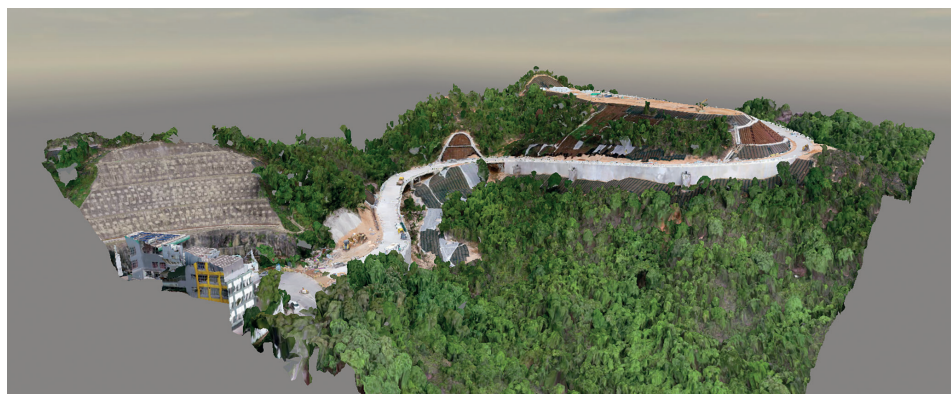
Photogrammetric Model of Portion 11 Generated from Point Cloud Data Image Courtesy of Drainage Services Department, HKSAR Government and AECOM Asia Company Limited and China State Construction Engineering (Hong Kong) Limited and MTECH Engineering Company Limited
