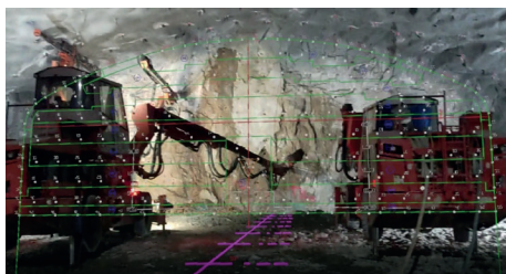
Drill Holes Verification from Trimble XR10 with HoloLens 2 Image Courtesy of Drainage Services Department, HKSAR Government and AECOM Asia Company Limited and China State Construction Engineering (Hong Kong) Limited and MTECH Engineering Company Limited
