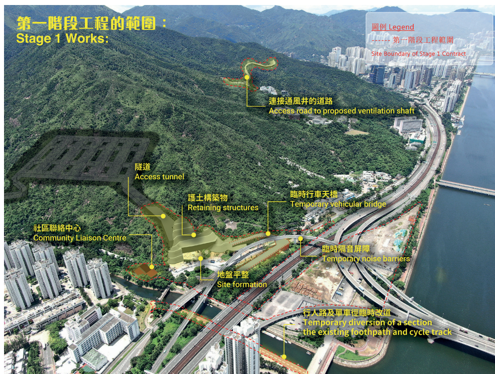
Relocation of Sha Tin Sewage Treatment Works to Caverns (Stage 1 Works) Overview Image Courtesy of Drainage Services Department, HKSAR Government and AECOM Asia Company Limited and China State Construction Engineering (Hong Kong) Limited and MTECH Engineering Company Limited
