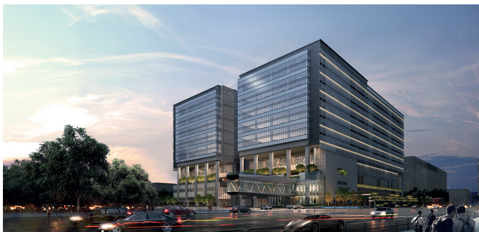
AMC is one of the first manufacture buildings to meet the industrial 4.0 standards. Image Courtesy of Gammon Construction Limited and Hong Kong Science and Technology Parks Corporation
