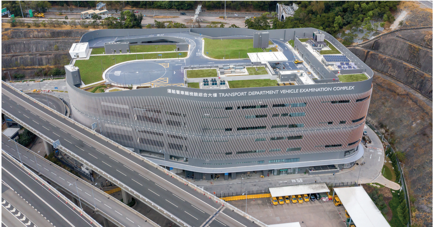
Design and Construction of Transport Department's Vehicle Examination Centre Image Courtesy of Hip Hing Engineering Company Limited and Architectural Services Department, HKSAR Government and Vircon Limited
