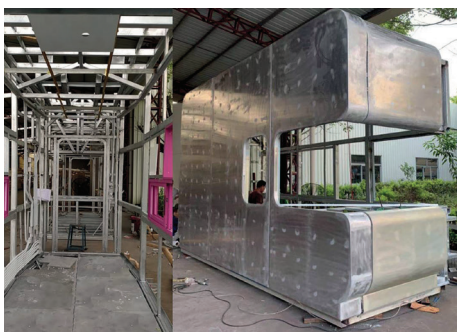
Off-site_MiC Prefabrication Image Courtesy of Hip Hing Engineering Company Limited and Architectural Services Department, HKSAR Government and Vircon Limited
