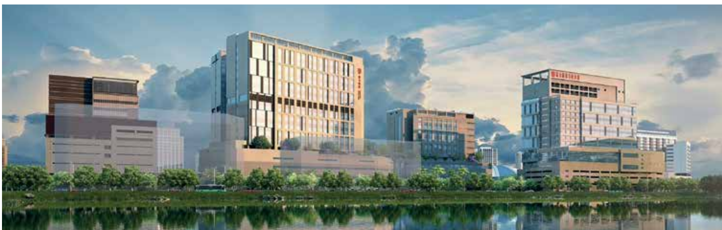
Island District Medical Complex, Macau Image Courtesy of China Construction Engineering (Macau) Company Limited
