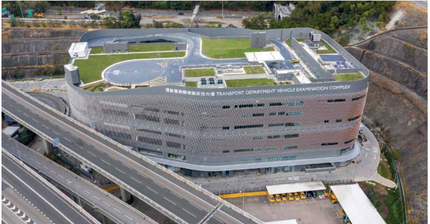
Design and Construction of Transport Department's Vehicle Examination Centre Image Courtesy of Hip Hing Engineering Company Limited and Architectural Services Department, HKSAR Government and Vircon Limited
