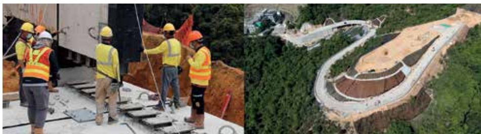
Lifting and assembly of retaining wall; Overview of retaining wall Image Courtesy of Drainage Services Department, HKSAR Government and AECOM Asia Company Limited
