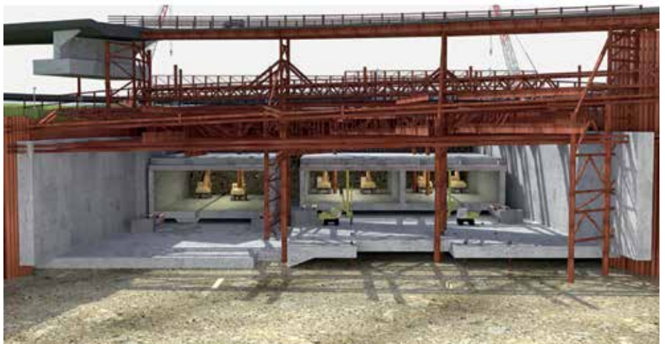
Simulation for construction sequence of box jacking Image Courtesy of Airport Authority Hong Kong and China State Construction Engineering (Hong Kong) Limited
