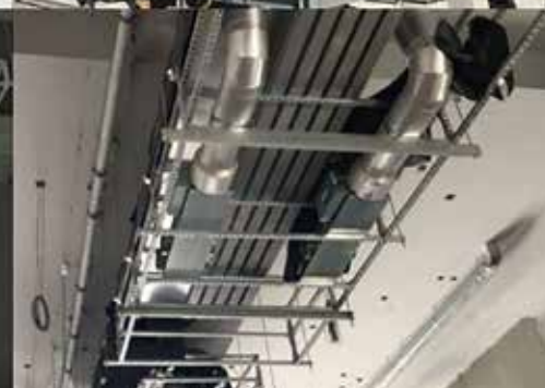
DfMA – Multi Trade integrated MEP (MiMEP) Image Courtesy of Hip Hing Engineering Company Limited and Architectural Services Department, HKSAR Government and Vircon Limited
