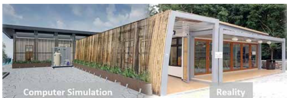
Computer Simulated Model of the Community Liaison Centre against the Reality Image Courtesy of Drainage Services Department, HKSAR Government and AECOM Asia Company Limited and China State Construction Engineering (Hong Kong) Limited and MTECH Engineering Company Limited
