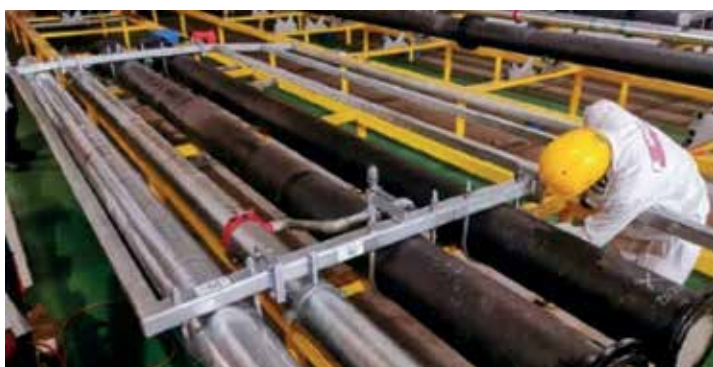
Modular Fabrication Factory Image Courtesy of Gammon Construction Limited
