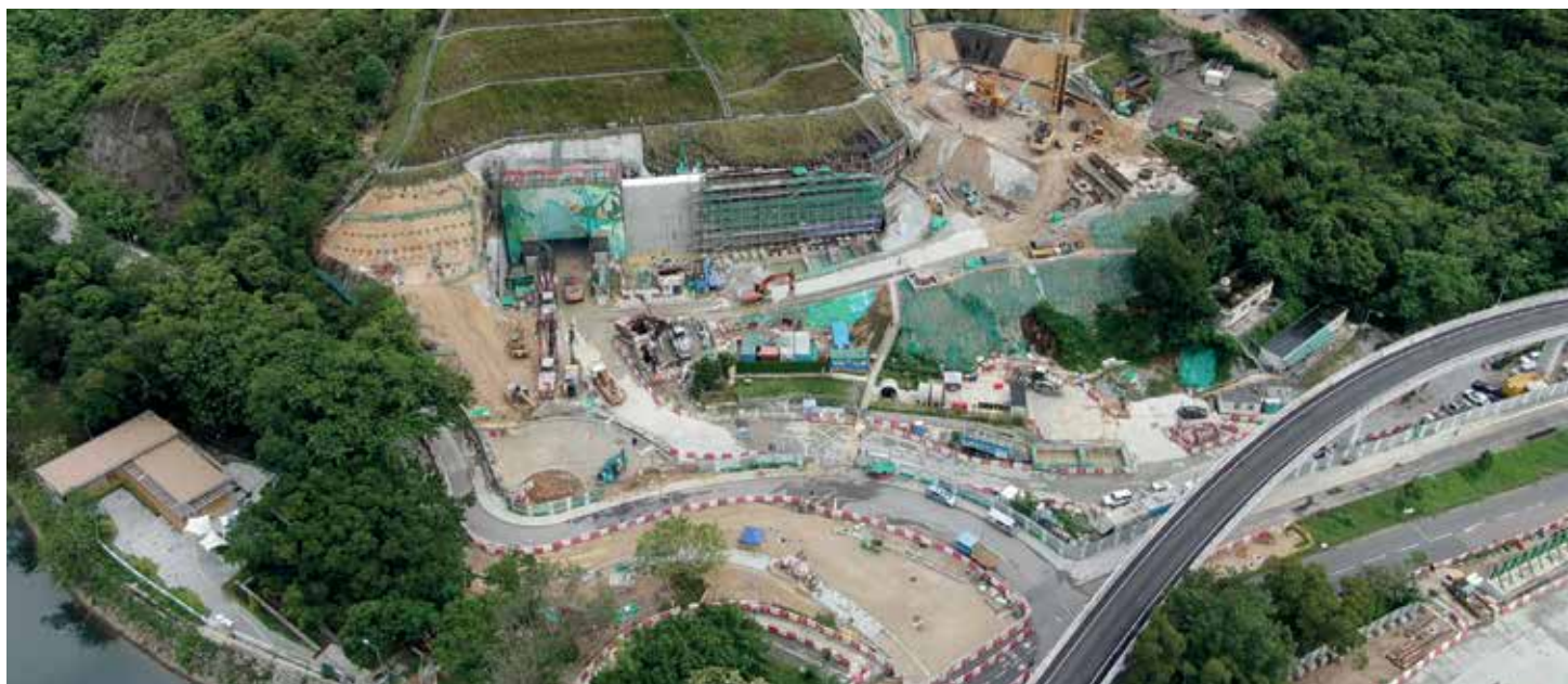
Site Photo of Relocation of Sha Tin Sewage Treatment Works to Caverns (Stage 1 Works)
