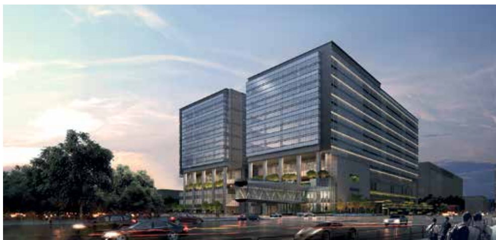
AMC is one of the first manufacture buildings to meet the industrial 4.0 standards. Image Courtesy of Gammon Construction Limited and Hong Kong Science and Technology Parks Corporation
