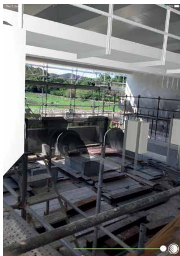
AR Application on Site Image Courtesy of Drainage Services Department, HKSAR Government and AECOM Asia Company Limited and The Jardine Engineering Corporation, Limited
