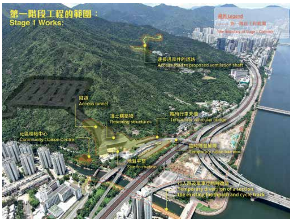
Relocation of Sha Tin Sewage Treatment Works to Caverns (Stage 1 Works) Overview Image Courtesy of Drainage Services Department, HKSAR Government and AECOM Asia Company Limited and China State Construction Engineering (Hong Kong) Limited and MTECH Engineering Company Limited
