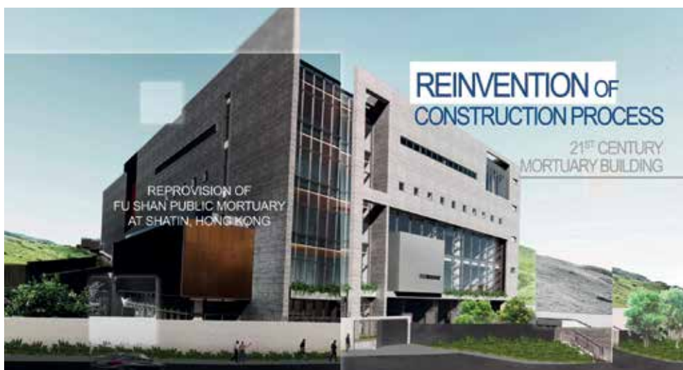
From BIM to DfMA: the reinvention of construction process of 21 st century mortuary building Image Courtesy of Architectural Services Department, HKSAR Government (ArchSD)
