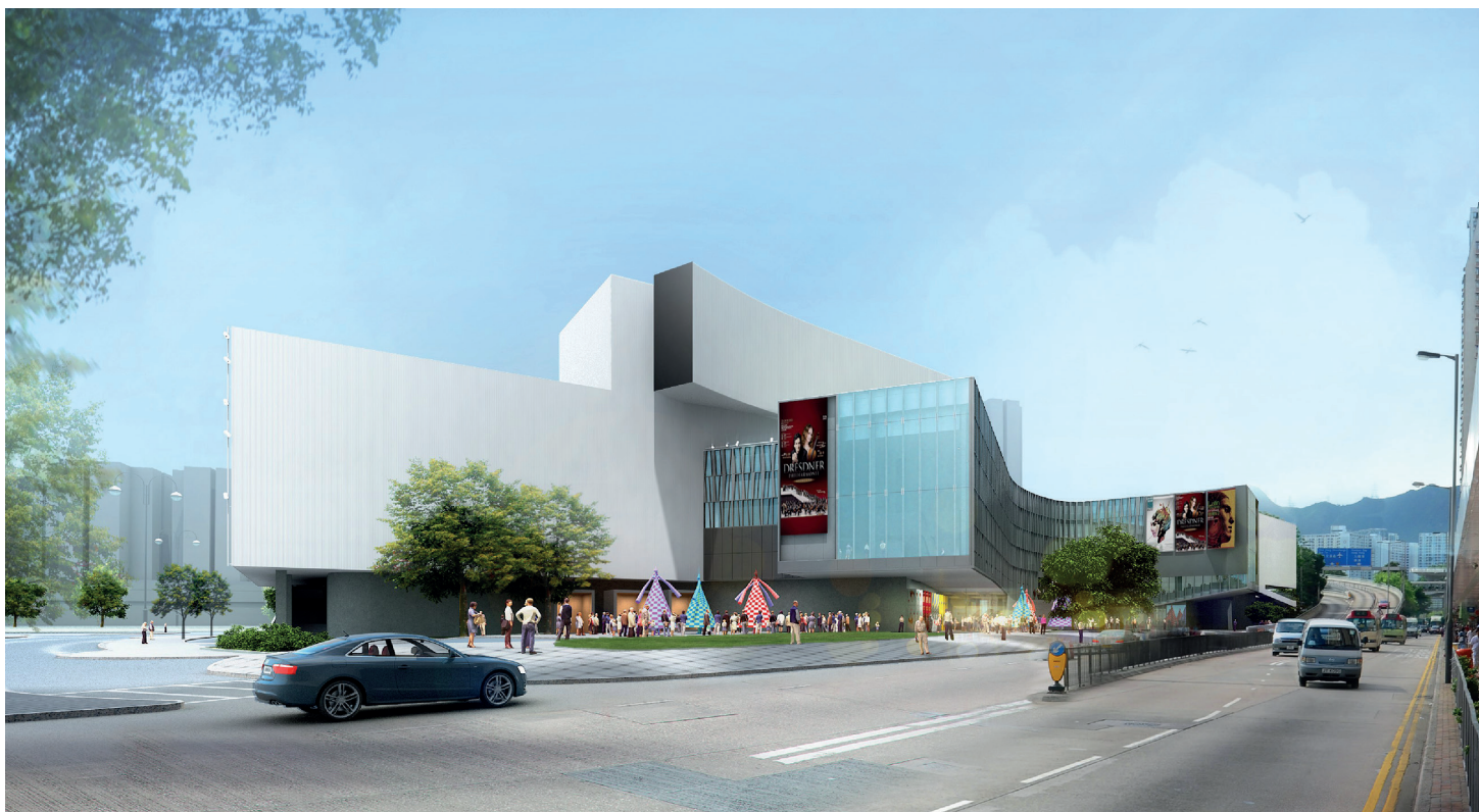
East Kowloon Cultural Centre external facade Image Courtesy of Leighton Contractors (Asia) Limited
