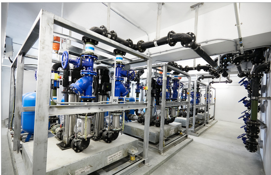
DfMA Water Pump Designed by BIM Image Courtesy of Architectural Services Department, HKSAR and China State Construction Engineering (Hong Kong) Limited and China State Construction International Medical Industry Development Company Limited
