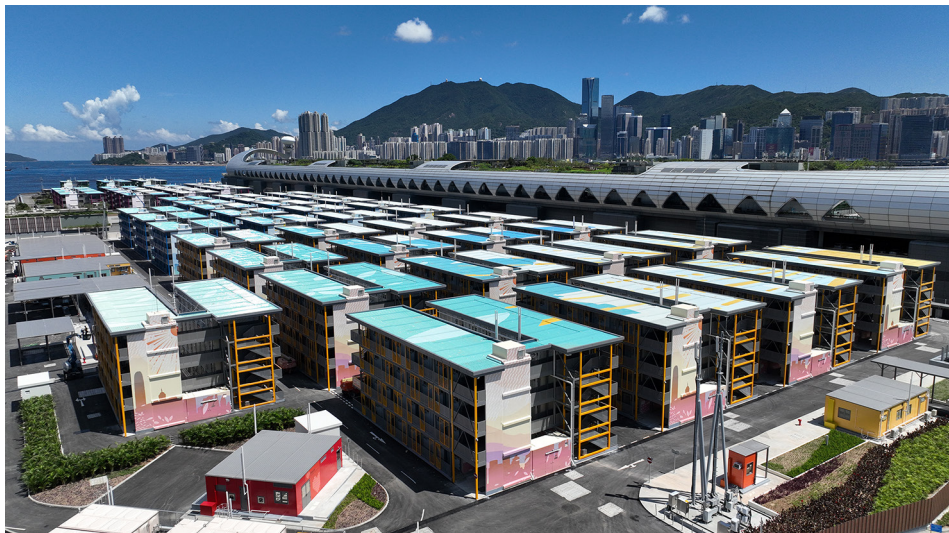
Graphic Design Works for KT Community Isolation Facility Image Courtesy of Architectural Services Department, HKSAR and China State Construction Engineering (Hong Kong) Limited and China State Construction International Medical Industry Development Company Limited
