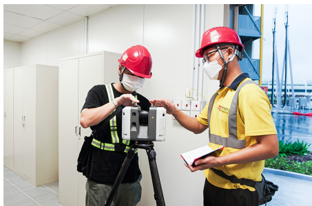
Laser Scan for BIM Model Checking Image Courtesy of Architectural Services Department, HKSAR and China State Construction Engineering (Hong Kong) Limited and China State Construction International Medical Industry Development Company Limited
