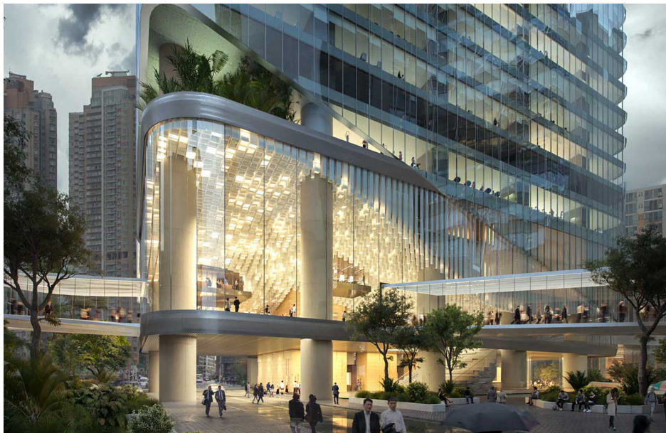
Jumbo Glass Panels spanning up to 15 meters Image Courtesy of Swire Properties Limited
