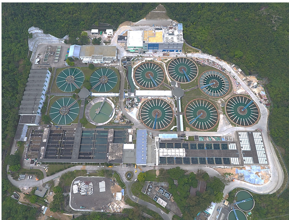
Initial Condition of STWTW Image Courtesy of Water Supplies Department, HKSAR Government and ATAL – Chun Wo – Ming Hing Joint Venture and Summit Technology (Hong Kong) Limited
