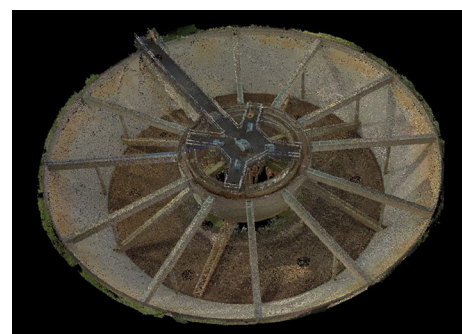
Point Cloud Image of Existing Clarifier Image Courtesy of Water Supplies Department, HKSAR Government and ATAL – Chun Wo – Ming Hing Joint Venture and Summit Technology (Hong Kong) Limited
