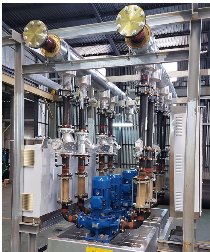
MiMEP Pump Module Image Courtesy of Electrical and Mechanical Services Department, HKSAR
