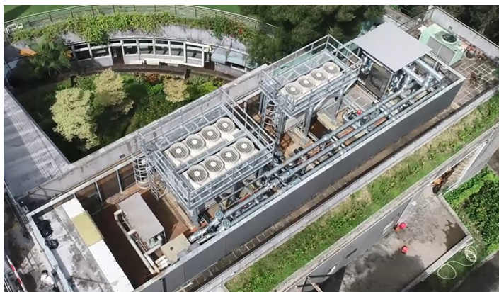
Project Completion Image Courtesy of Electrical and Mechanical Services Department, HKSAR
