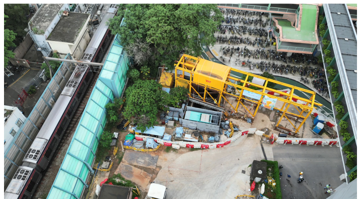
TBM Launching Pit near Sheung Shui MTR Station Image Courtesy of Water Supplies Department, HKSAR Government
