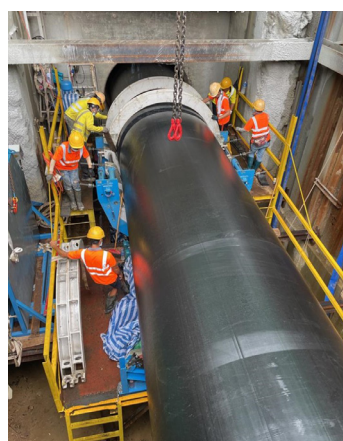
Lifting and aligning of OD2000 PE pipes for butt fusion welding Image Courtesy of Water Supplies Department, HKSAR Government
