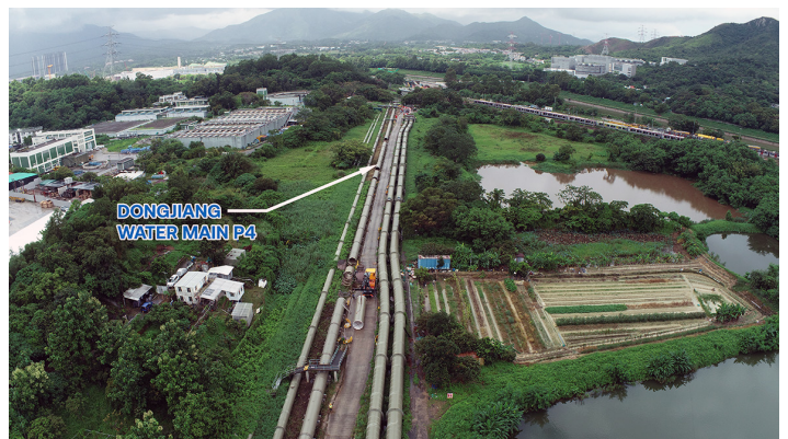
Replacement of Exposed DongJiang Water Main P4 Image Courtesy of Water Supplies Department, HKSAR Government
