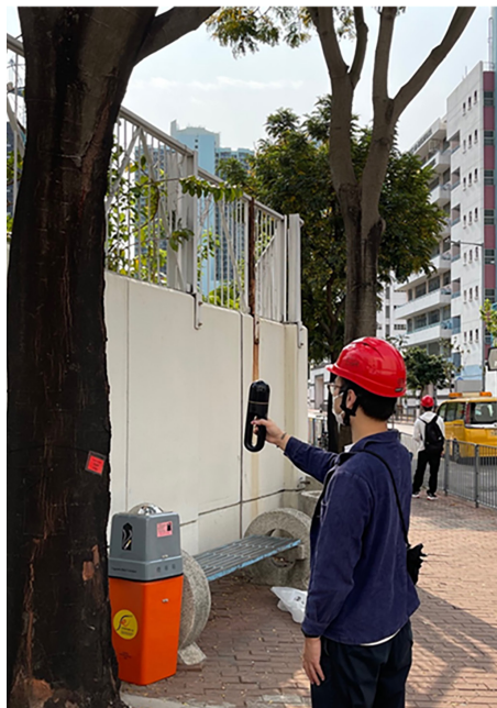
Leica Handheld Scanner for conducting 3D scanning works. Image Courtesy of Architectural Services Department, HKSAR and Shui On Joint Venture
