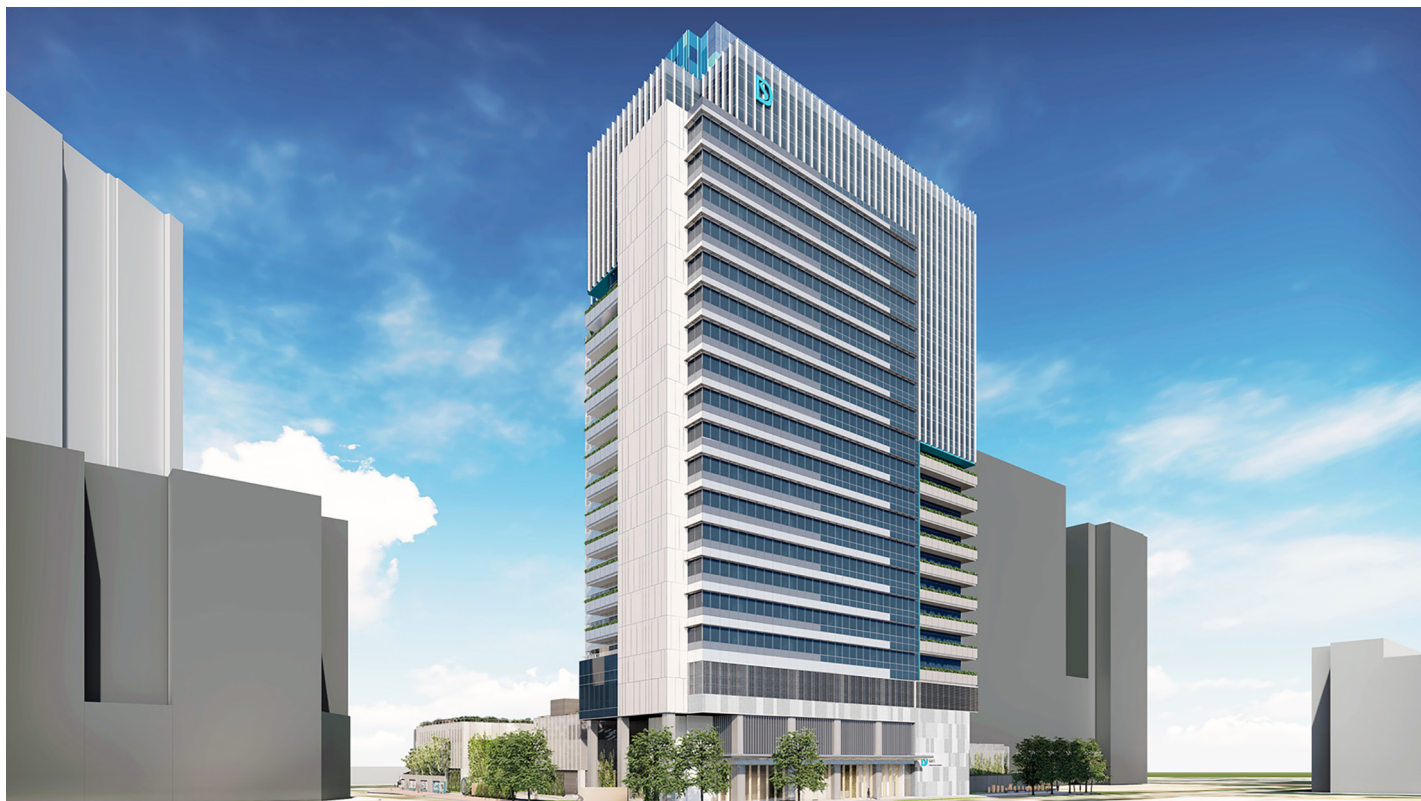
Overall view of DSD Building. Image Courtesy of Architectural Services Department, HKSAR and Shui On Joint Venture
