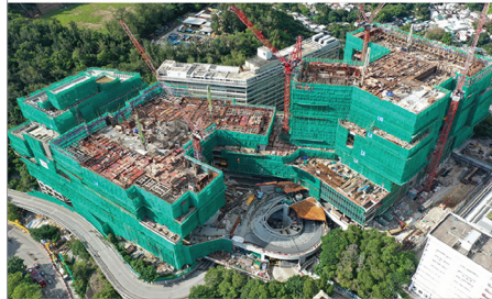
4-D BIM provided clear pictures of site conditions for bamboo scaffolding planning. Image Courtesy of Architectural Services Department, HKSAR and Shui On Joint Venture and WSP Hong Kong Limited
