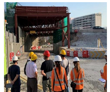
Site discussion before removal
