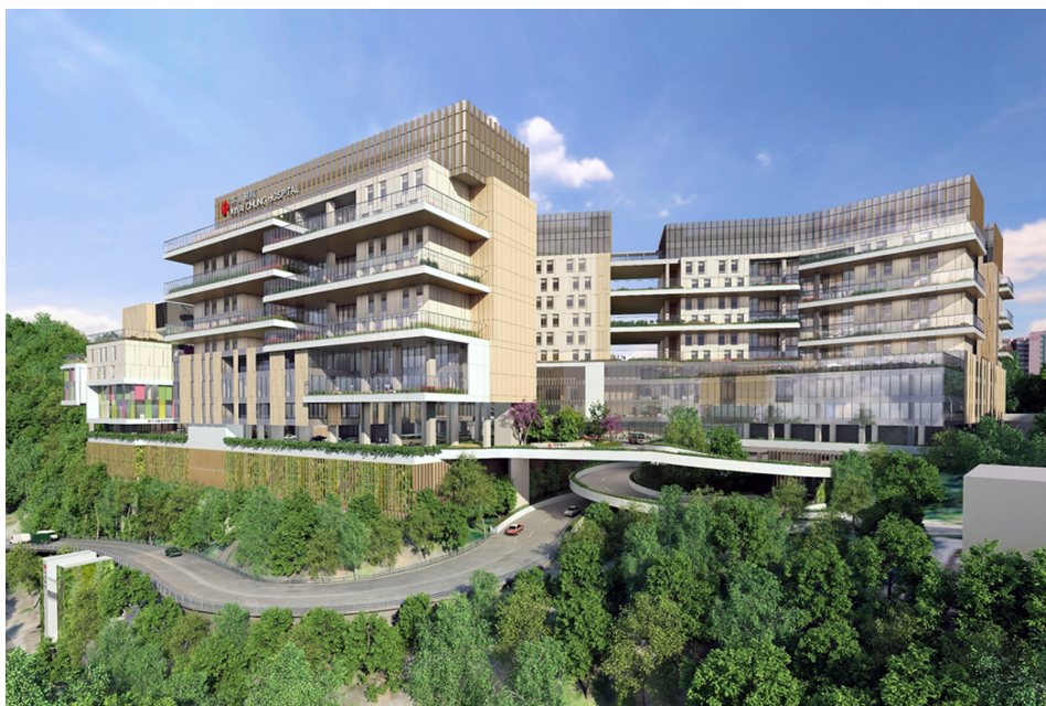
Redevelopment of Kwai Chung Hospital - creating a supportive environment for patient-focused mental healthcare Image Courtesy of Architectural Services Department, HKSAR and Shui On Joint Venture and WSP Hong Kong Limited
