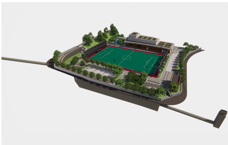
Overall View of the Sau Nga Road Stormwater Storage Scheme with Re-provisioned Sau Nga Road Playground Image Courtesy of Drainage Services Department, HKSAR Government and Kwan Lee - Chun Wo Joint Venture and Blue BIM Limited
