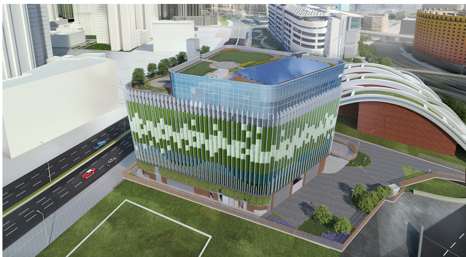
Bird's eye view of Additional District Cooling Plant Image Courtesy of Paul Y. - Qianhai Joint Venture and Vircon Limited
