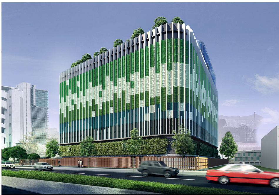
Additional District Cooling Plant Image Courtesy of Paul Y. - Qianhai Joint Venture and Vircon Limited
