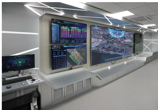
NAH on Site C-Smart Center Image Courtesy of China State Construction Engineering (Hong Kong) Limited
