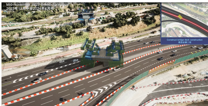
Simulation of form traveller operation for bridge construction at Fanling Highway Image Courtesy of Civil Engineering and Development Department, HKSAR Government and AECOM Asia Company Limited and CRCC - Paul Y. Joint Venture and Tyfron Consultancy Limited
