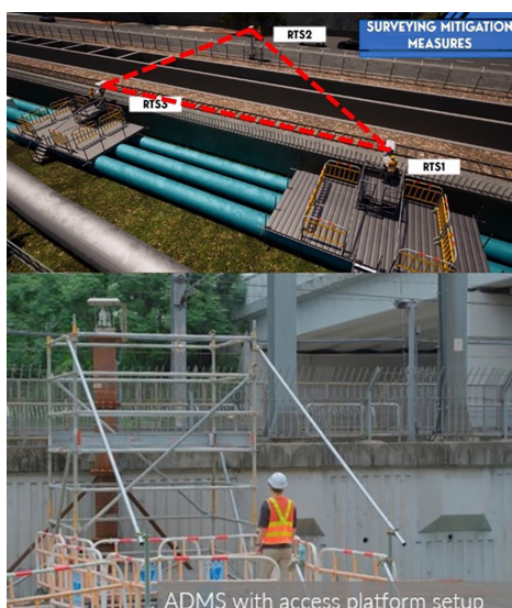
BIM Analysis for the Optimum Position of ADMS Monitoring Points Image Courtesy of WSD and Atkins and CWE and TYFRON
