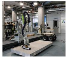
Fig. 3 One sheet of cement backer board being placed in the spandrel panel assembly
