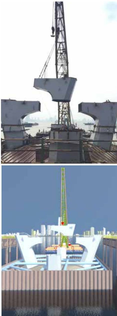
图18 Autodesk Navisworks 桥塔节段吊装与现场对比
