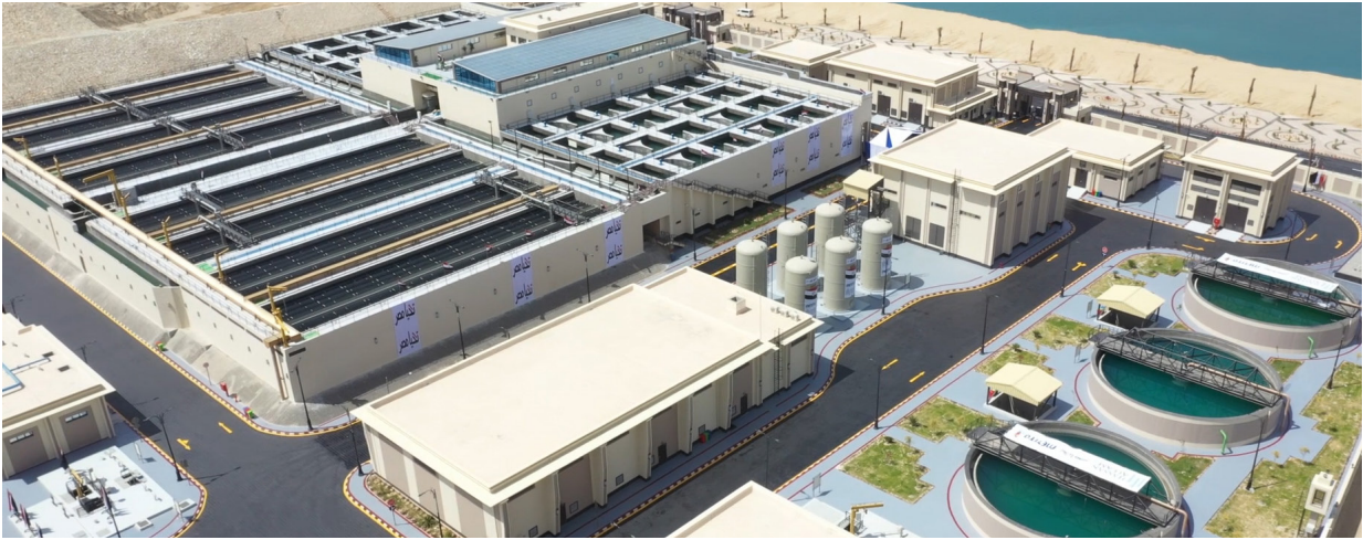
Al Mahsama agricultural drainage treatment, recycling and reuse plant in Al-Ismailia, Egypt
