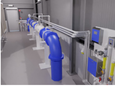
Water Treatment Works Coagulation Dosing Gallery
