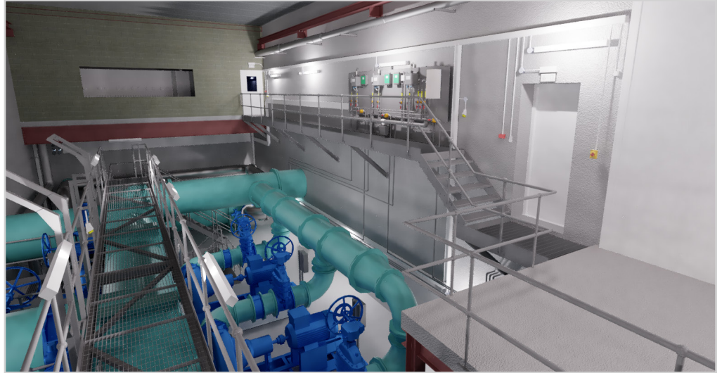
Water Treatment Works Transfer Pump Station
