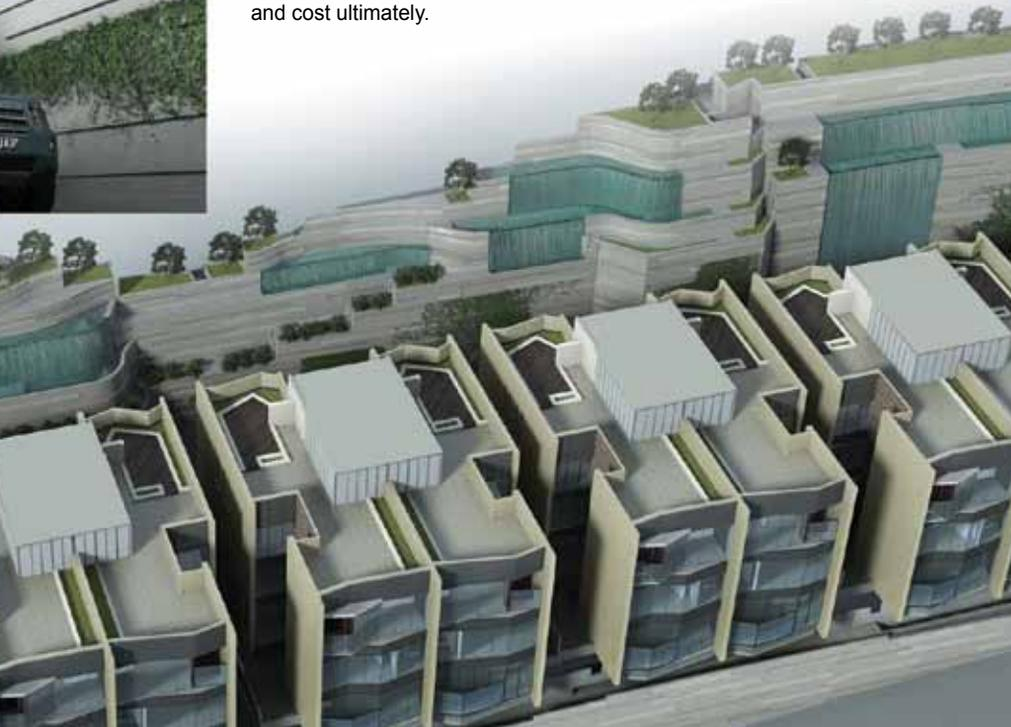
was significantly over budget. The project team worked to streamline the design in the BIM model, and within a month achieved a 40% reduction in the concrete volume and formwork needed.
