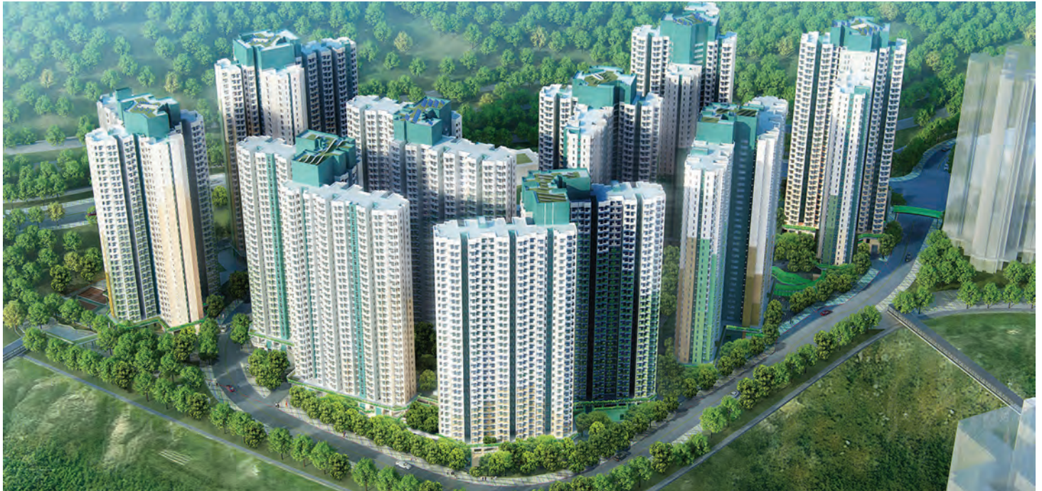
Image courtesy of Hong Kong Housing Authority
