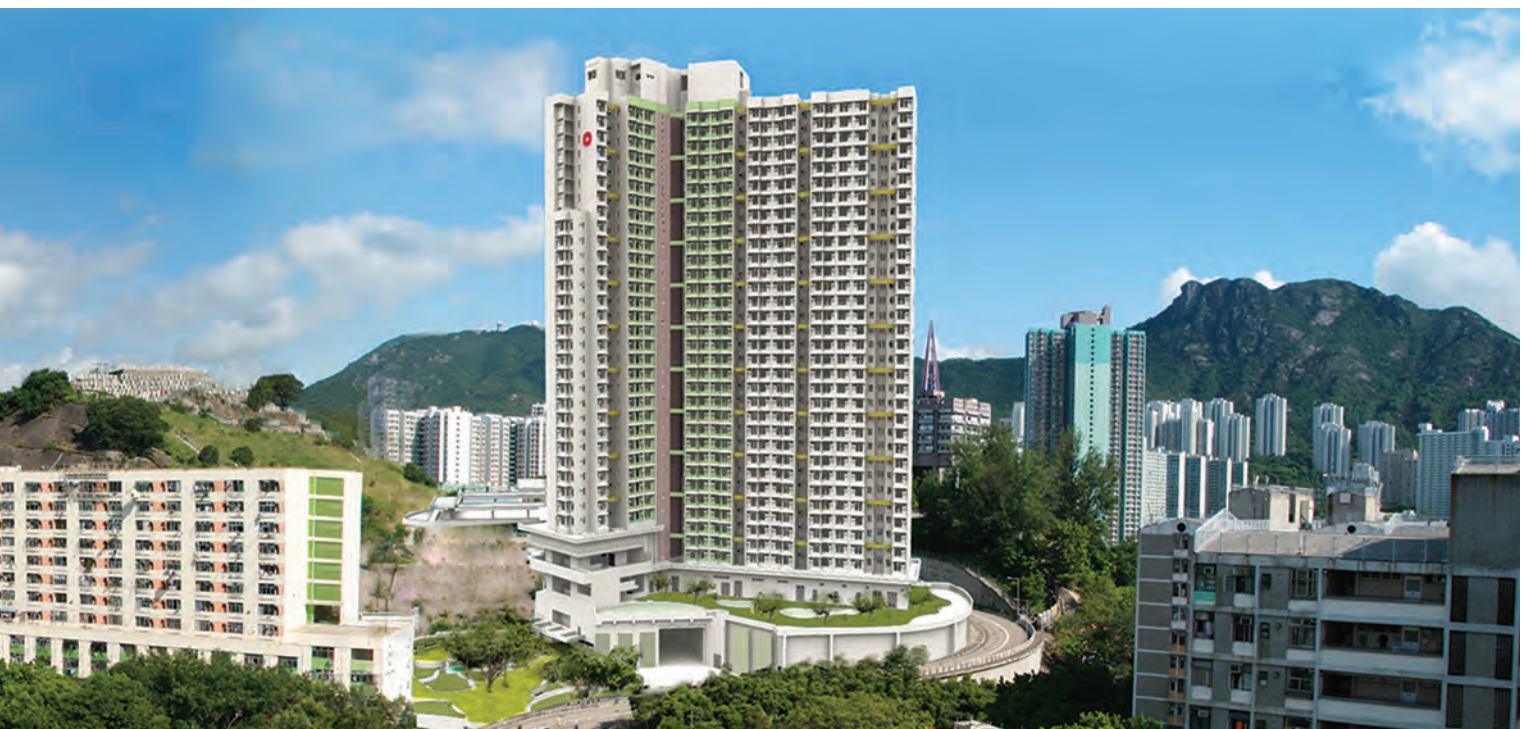
Image courtesy of Hong Kong Housing Authority
