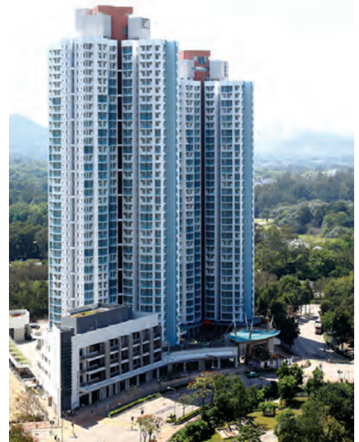
Image courtesy of Hong Kong Housing Authority
