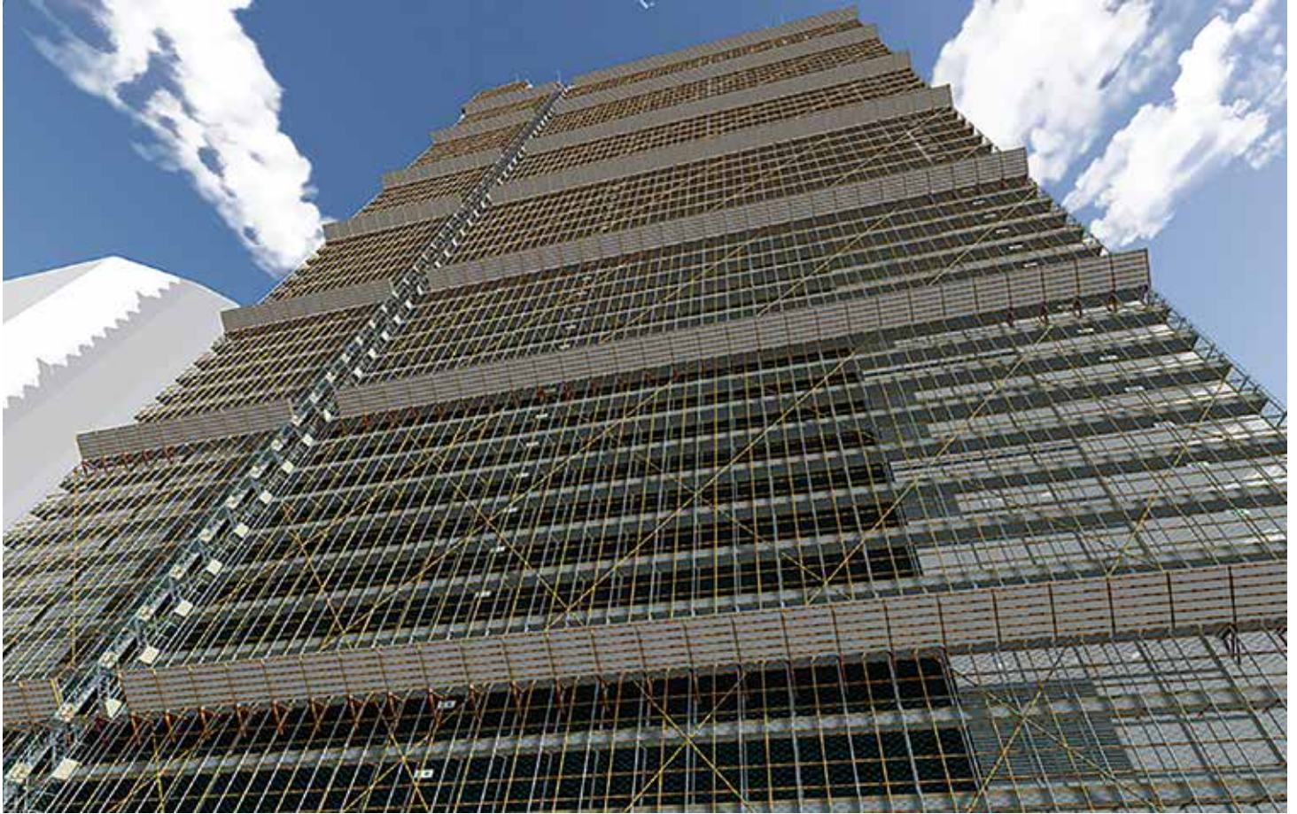
Bottom view of CLP Shatin Centre (with Bamboo Scaffolding) in BIM Image courtesy of CLP Power Hong Kong Limited
