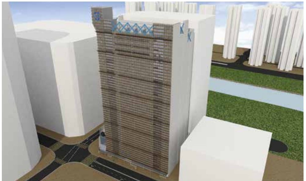
General view of CLP Shatin Centre (with Bamboo Scaffolding) in BIM Image courtesy of CLP Power Hong Kong Limited
