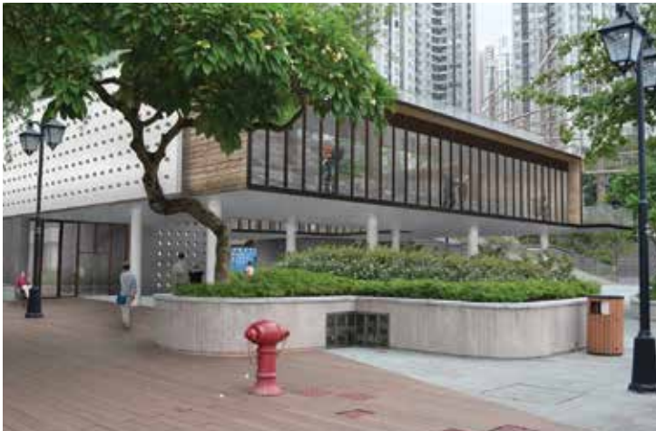
In early design stage, traditional photo montage was composed by architect to highlight the impression of the project Image courtesy of Architectural Services Department, HKSAR Government
