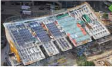
Overview site progress of roof construction.
