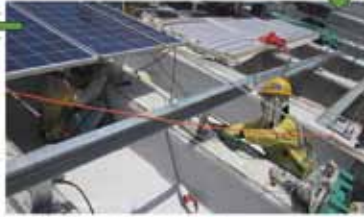
Assemble PV panels on curvy roof on site.
