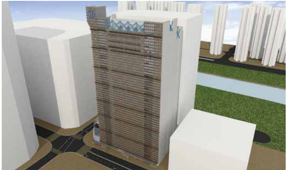
General view of CLP Shatin Centre (with Bamboo Scaffolding) in BIM Image courtesy of CLP Power Hong Kong Limited
