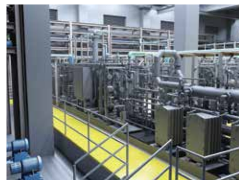
On-site Chlorine Generation Skids with Walkways for Operation and Maintenance Access Fitted within Chlorine Store using BIM Model to Optimize Space Utilization Image courtesy of Water Supplies Department, HKSAR Government
