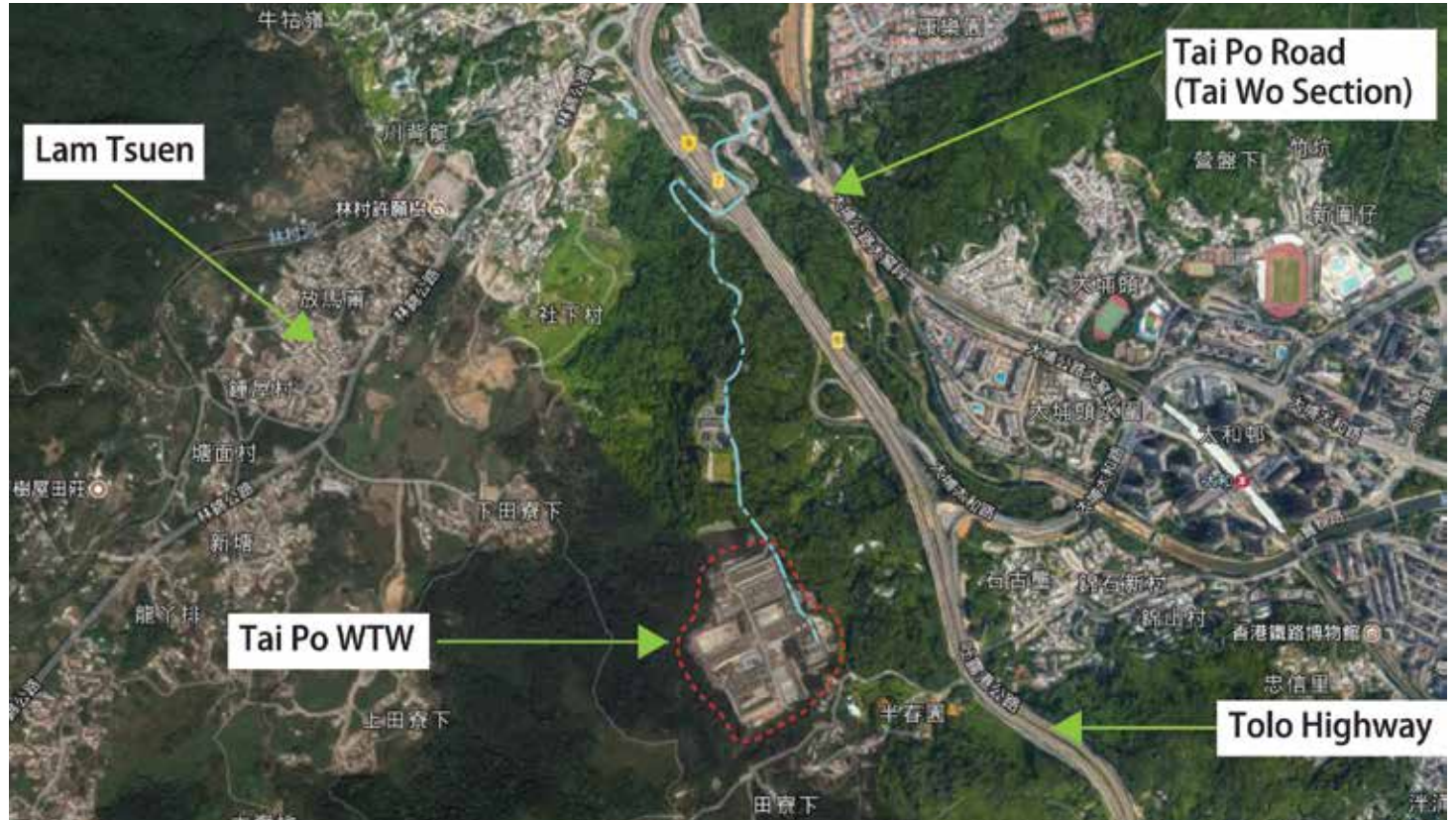
Tai Po Water Treatment Works Located on a Hilltop Overlooking Tai Po Urban and Rural Developments Image courtesy of Water Supplies Department, HKSAR Government
