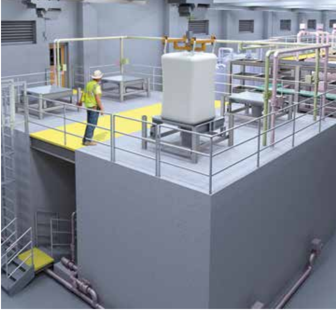
Visualization of the Access Provided for Operation and Maintenance of Salt Loading Facilities and Brine Tanks Image courtesy of Water Supplies Department, HKSAR Government
