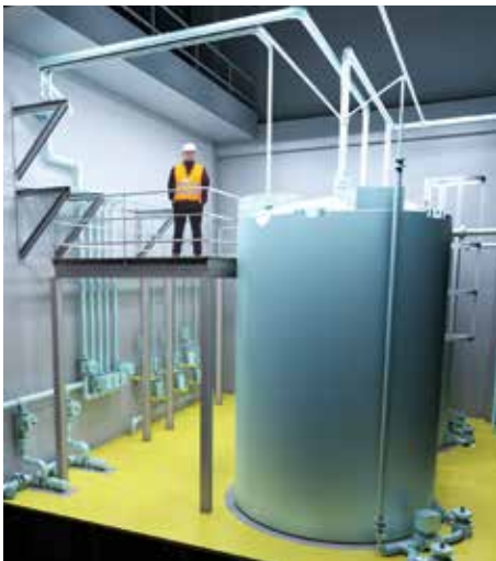
Visualization of the Elevated Maintenance Access of Hypochlorite Storage Tanks and Dosing facilities Image courtesy of Water Supplies Department, HKSAR Government
