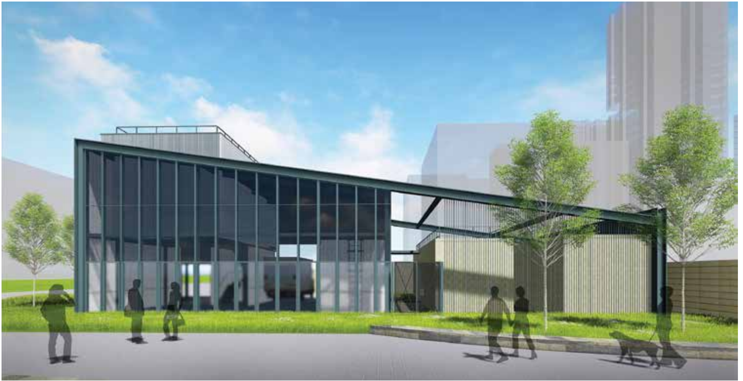
The Kai Tak RCP is constructed mainly by steel structure and designed with glass, masonry block and vertical green as external façade. Image courtesy of Architectural Services Department, HKSAR Government
