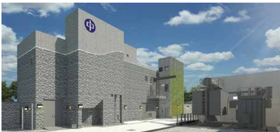
BIM enhances the multidisciplinary collaboration. The configuration is optimised for installation of high voltage plant equipment Image courtesy of CLP Power Hong Kong Limited
