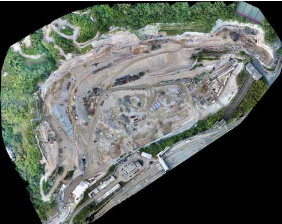
Terrain model by drone to increase accuracy and reduced survey time of existing site condition Image courtesy of Civil Engineering and Development Department, HKSAR Government and AECOM Asia Company Limited and Leighton-China State Joint Venture
