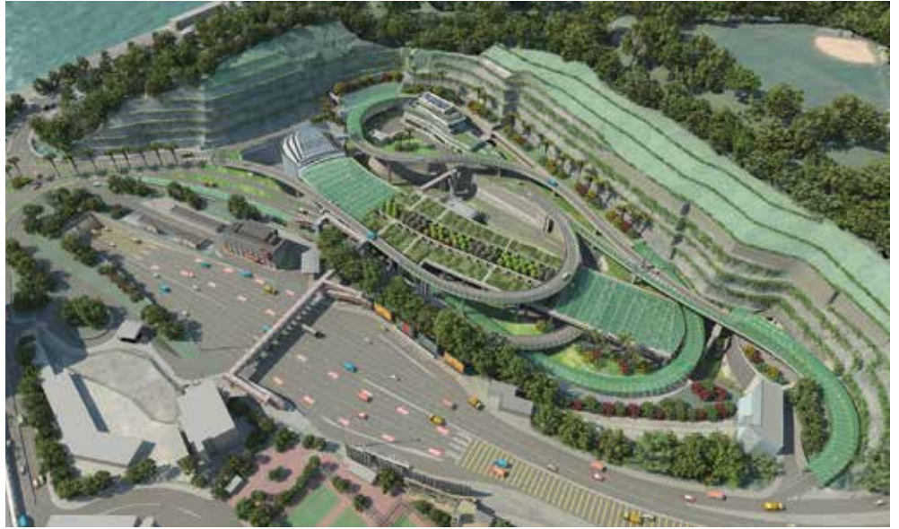
Aerial view of Lam Tin Interchange Image courtesy of Civil Engineering and Development Department, HKSAR Government and AECOM Asia Company Limited and Leighton-China State Joint Venture
