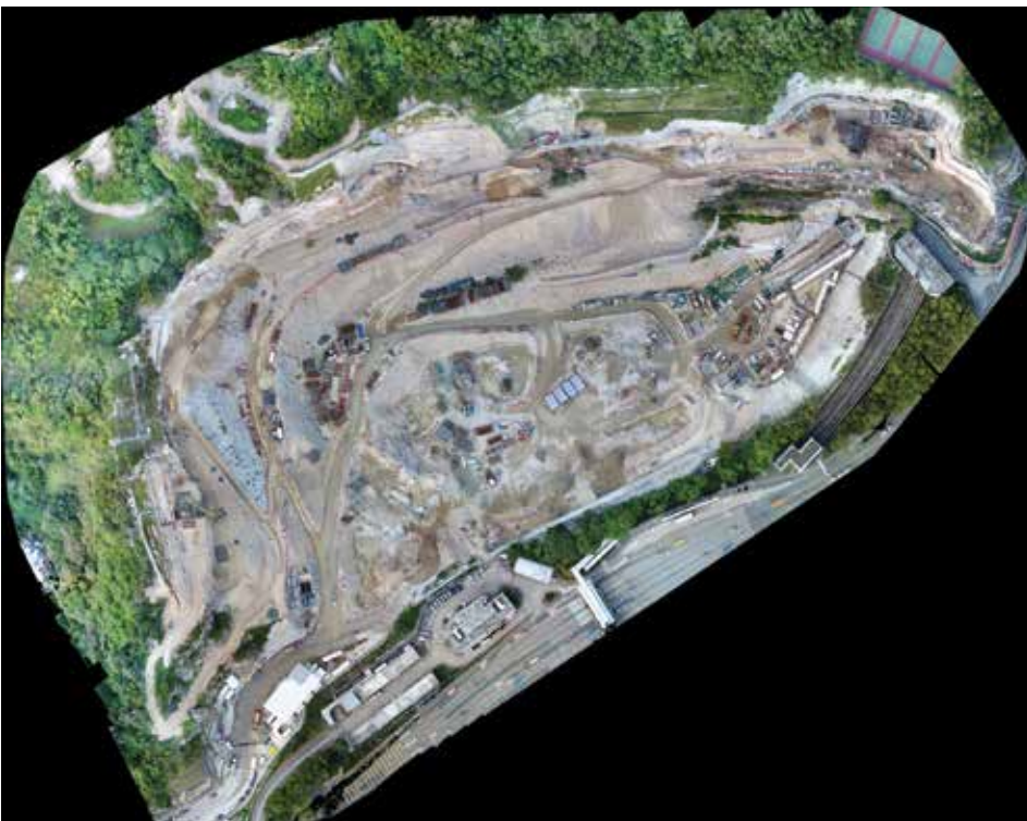
Terrain model by drone to increase accuracy and reduced survey time of existing site condition Image courtesy of Civil Engineering and Development Department, HKSAR Government and AECOM Asia Company Limited and Leighton-China State Joint Venture
