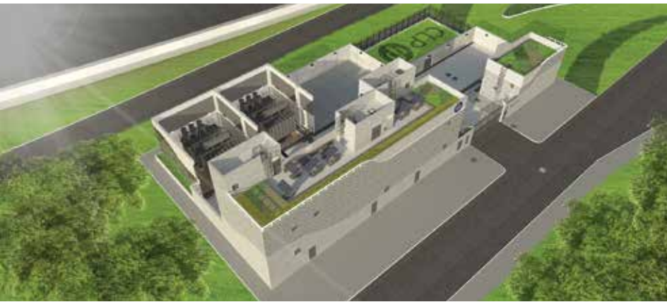
Visualisation of the aerial view of the substation Image courtesy of CLP Power Hong Kong Limited
