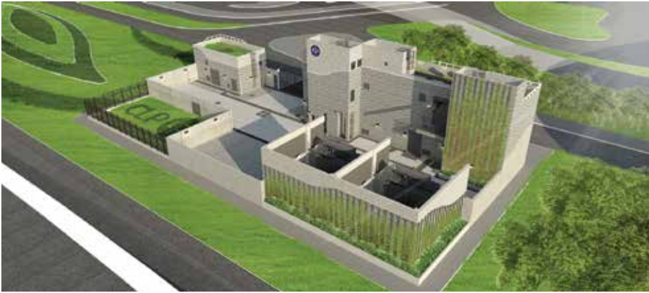
Visualisation of the aerial view of the substation Image courtesy of CLP Power Hong Kong Limited
