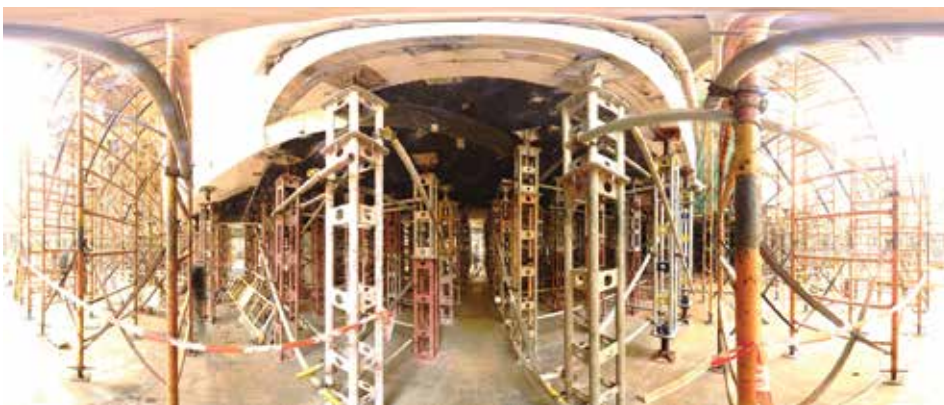
Planning of Temporary Propping via 3D Laser Scanning Image courtesy of Hip Hing Construction Company Limited
