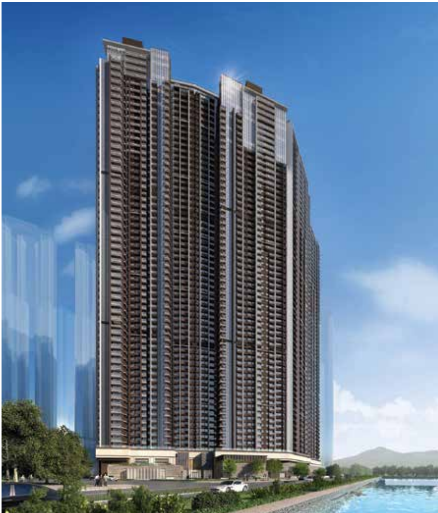
Overall view of Lohas Park Phase 6 at Tseung Kwan O Image courtesy of Nan Fung Development Limited
