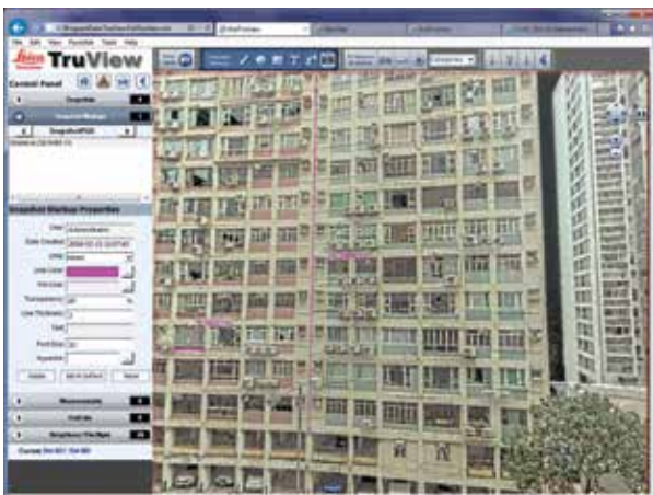
We use point cloud to fast check the building condition with existing structure and facilities Image courtesy of Urban Renewal Authority
