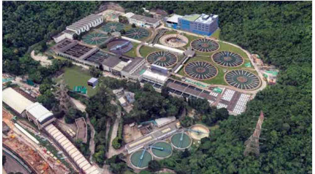
General View of the Sha Tin Water Treatment Works after Project Completion Image courtesy of Water Supplies Department, HKSAR Government and Ming Hing – Ming Hing Civil – Vasteam Joint Venture and Summit Technology (Hong Kong) Limited
