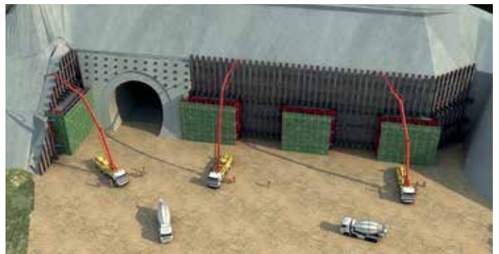
Construction Simulation of Retaining Walls of Tunnel Portal Image Courtesy of Drainage Services Department, HKSAR Government and AECOM Asia Company Limited and China State Construction Engineering (Hong Kong) Limited and MTECH Engineering Company Limited
