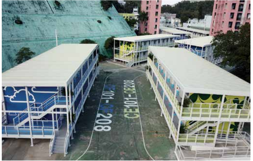
Site Photo of Pat Heung Quarantine Centre Image Courtesy of Hip Hing Engineering Company Limited and Architectural Services Department, HKSAR Government
