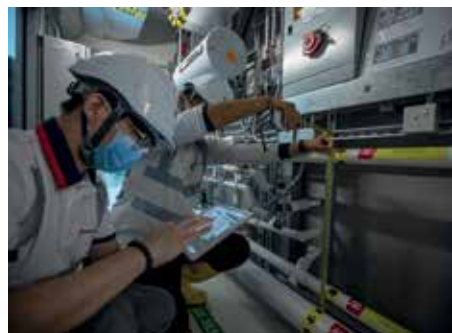
BIM As-Built Verification Image Courtesy of Gammon Engineering & Construction Company Limited
