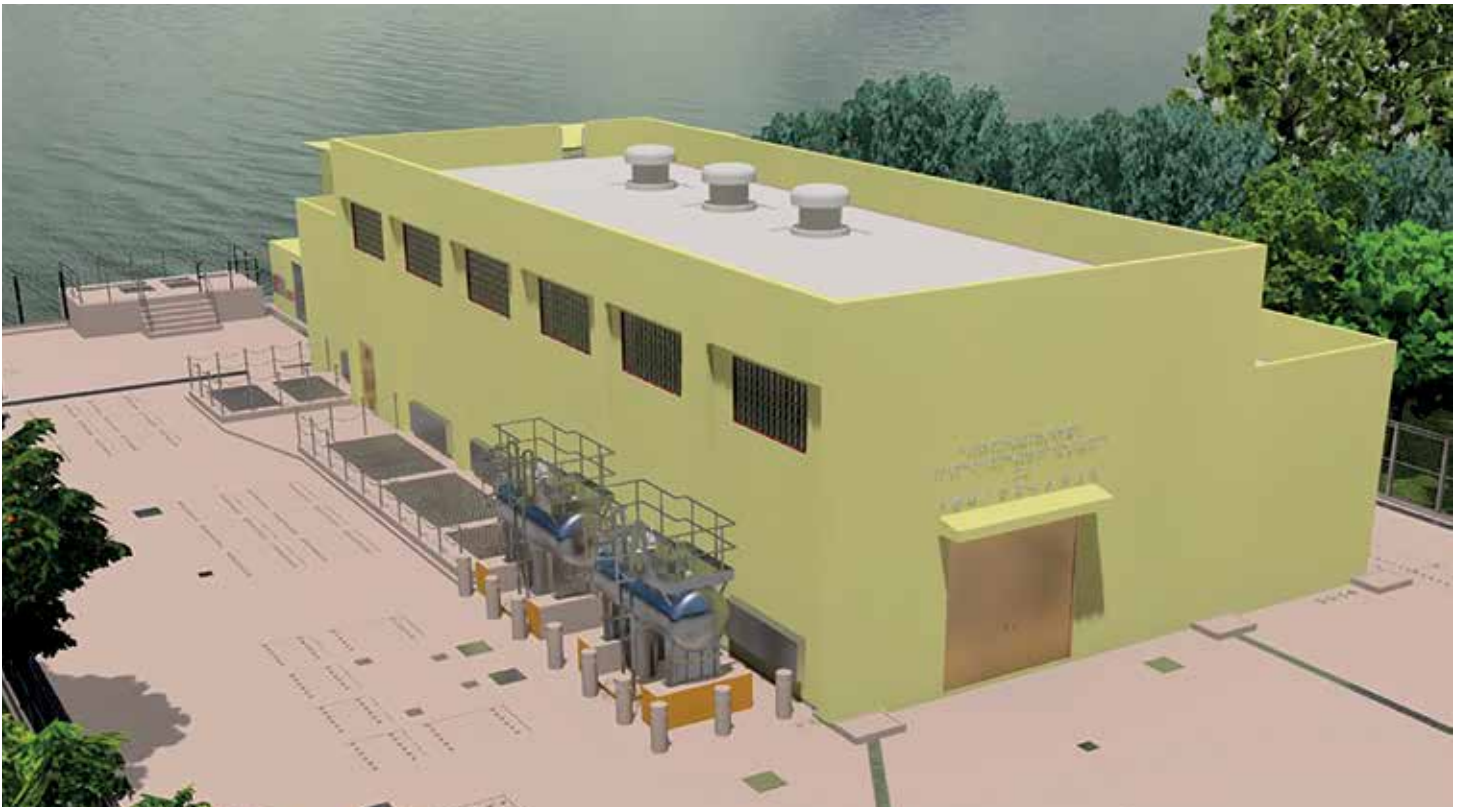
Overview of the Siu Sai Wan Salt Water Pumping Station Image Courtesy of Water Supplies Department, HKSAR Government
