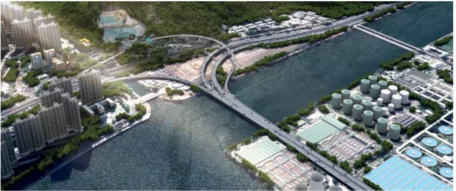
Relocation of Sha Tin Sewage Treatment Works to Caverns – Site Preparation and Access Tunnel Construction Image Courtesy of Drainage Services Department, HKSAR Government and AECOM Asia Company Limited and China State Construction Engineering (Hong Kong) Limited and MTECH Engineering Company Limited
