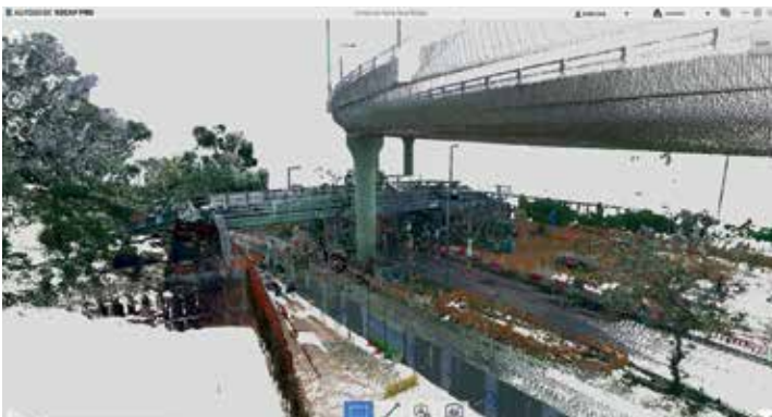
Point Cloud Scanning of Temporary Vehicular Steel Bridge Image Courtesy of Drainage Services Department, HKSAR Government and AECOM Asia Company Limited and China State Construction Engineering (Hong Kong) Limited and MTECH Engineering Company Limited
