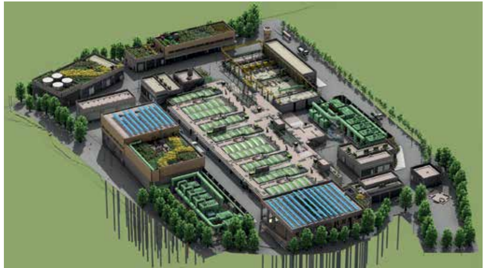
Site View of San Wai Sewage Treatment Works Image Courtesy of Drainage Services Department, HKSAR Government and AECOM Asia Company Limited and ATAL-Degremont-China Harbour Joint Venture
