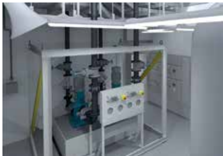
Modularized plant room facilitate to achieve just in time installation. Image Courtesy of Global Switch
