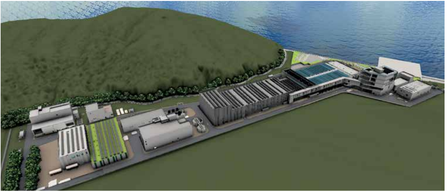
TKO Desalination Plant Overall View
