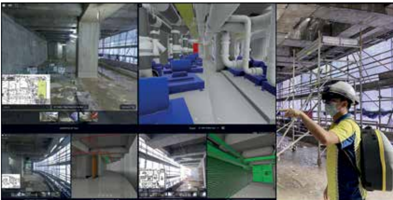
Site Condition and BIM Model Comparison by MR Equipment and Panoramagram Image Courtesy of Yee Fai Construction Company Limited
