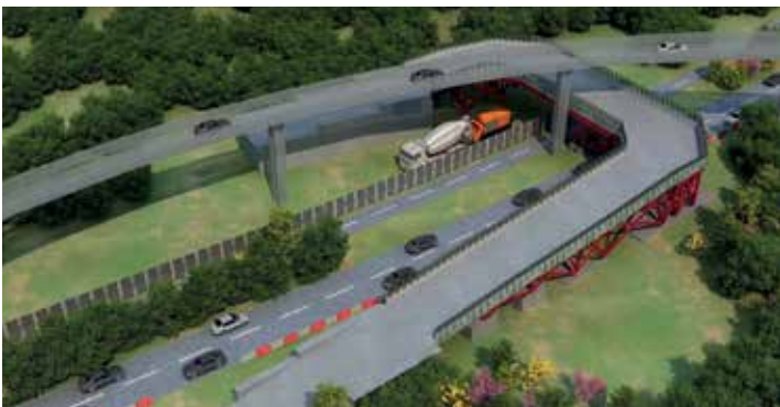
Design for Manufacture and Assembly (DfMA) of Temporary Vehicular Steel Bridge Image Courtesy of Drainage Services Department, HKSAR Government and AECOM Asia Company Limited and China State Construction Engineering (Hong Kong) Limited and MTECH Engineering Company Limited
