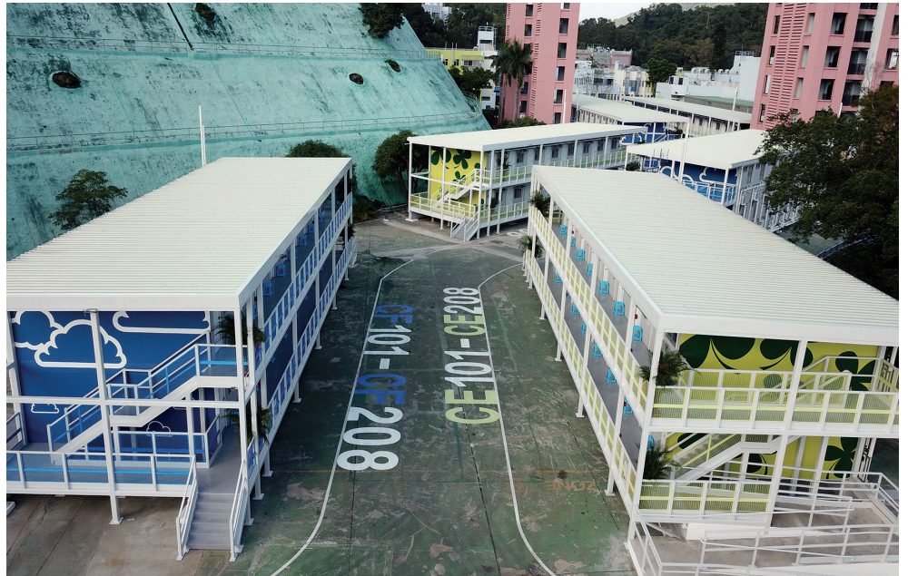
Site Photo of Pat Heung Quarantine Centre Image Courtesy of Hip Hing Engineering Company Limited and Architectural Services Department, HKSAR Government
