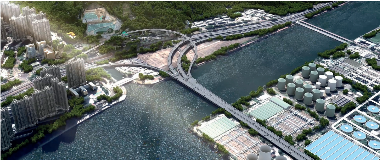
Relocation of Sha Tin Sewage Treatment Works to Caverns – Site Preparation and Access Tunnel Construction Image Courtesy of Drainage Services Department, HKSAR Government and AECOM Asia Company Limited and China State Construction Engineering (Hong Kong) Limited and MTECH Engineering Company Limited
