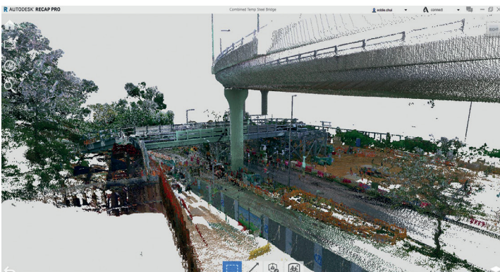
Point Cloud Scanning of Temporary Vehicular Steel Bridge Image Courtesy of Drainage Services Department, HKSAR Government and AECOM Asia Company Limited and China State Construction Engineering (Hong Kong) Limited and MTECH Engineering Company Limited
