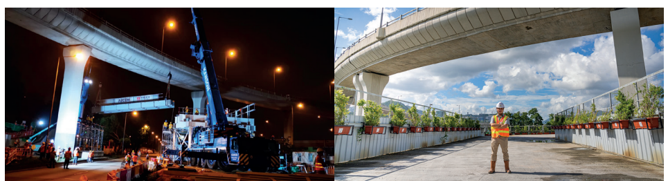
Lifting of the bridge deck segments at night and completed steel bridge Image Courtesy of Drainage Services Department, HKSAR Government and AECOM Asia Company Limited
