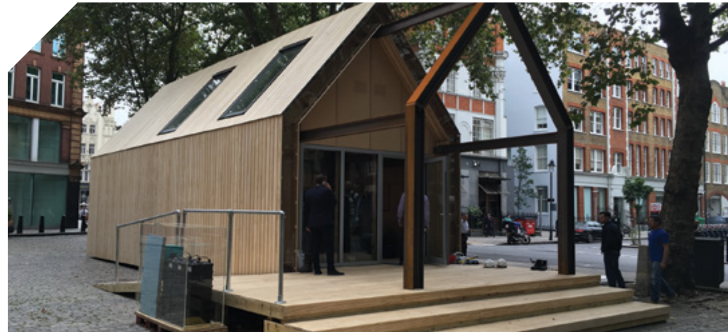
The Circular House, built with “borrowed” materials to be returned after disassembly. Courtesy BAM.
