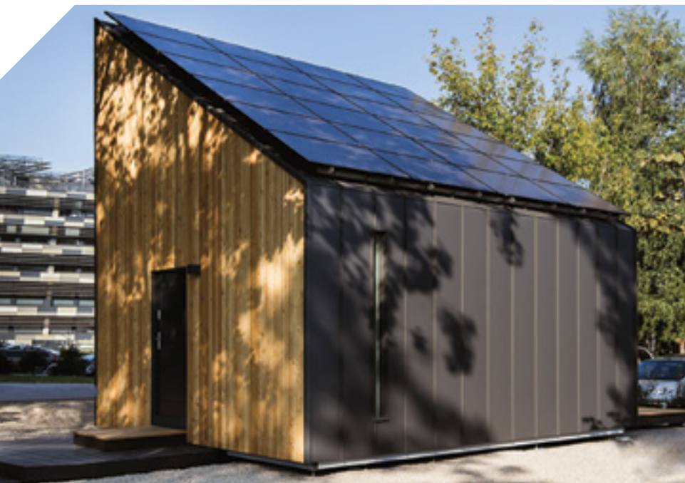
For a typical European climate, the Solace House's array of 24 solar panels can produce slightly more energy in a year than the homeowners will use. Courtesy Solace House.
