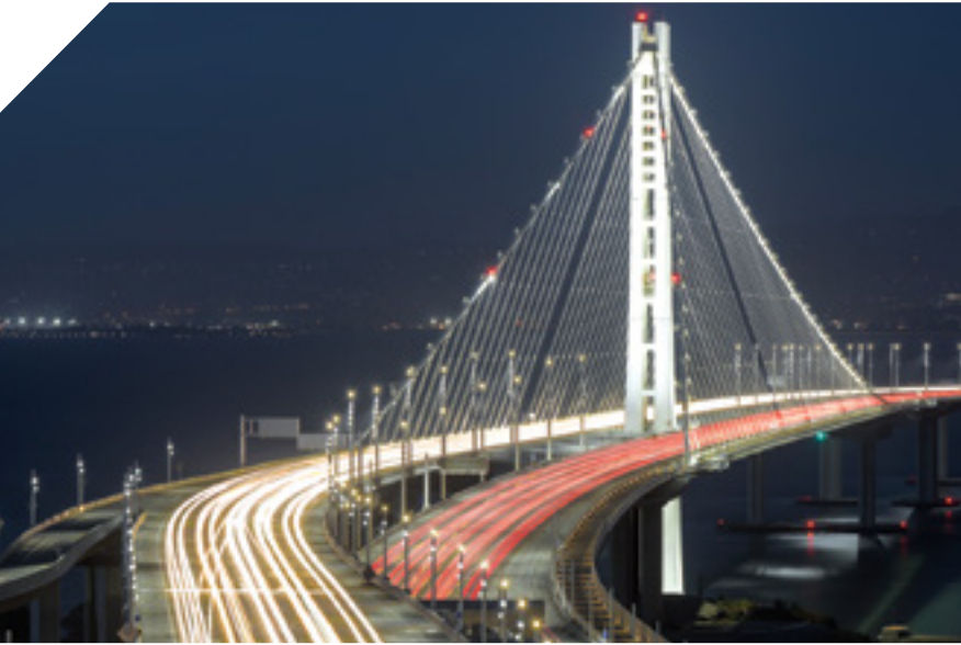
Computer simulations showed how “accordion-style” expansion joints and other seismic innovations would absorb earthquake shocks on the new eastern span of the Bay Bridge.
