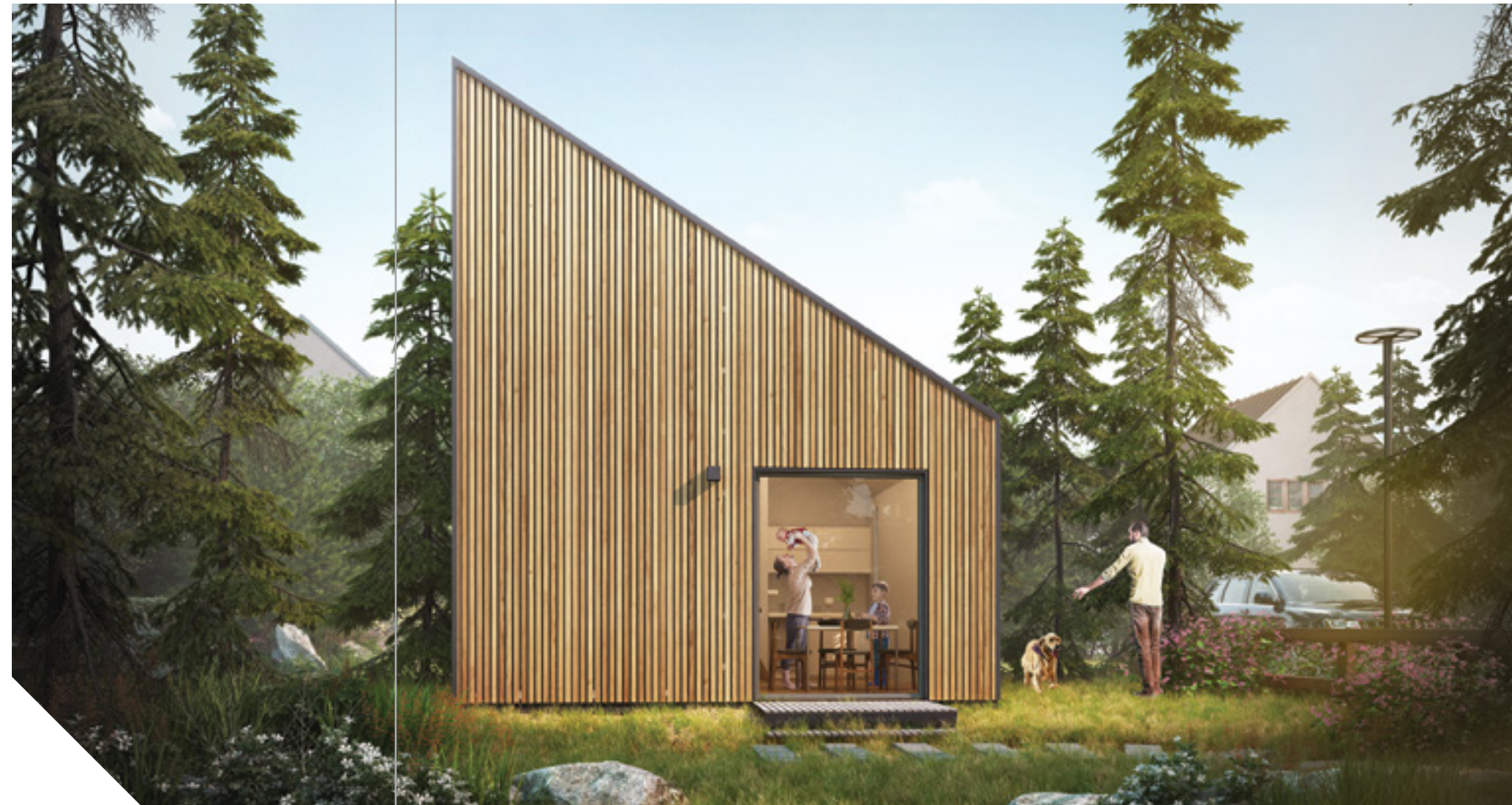
The prefabricated Solace house can travel in a single cargo container and takes about three days to assemble with a crew of three people. Courtesy Solace House.
